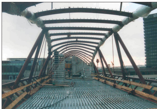
Fig. 2: Primary structure of 7 th floor office space
